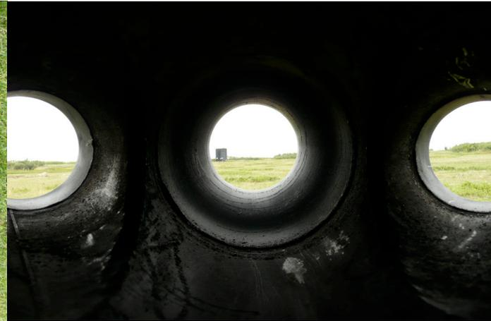
THE OUTER PORTS OF THE STINGMASTER ARE ARRANGED AT ANGLES SUCH THAT THE PRESSURE TUBE PASSING INTO THE TANK PASSES OVER A FIRST SECTION OF TANK FLOOR AND THE NEXT PORTS ALLOW PASSAGE OVER THE SECOND SECTION AND THIRD SECTION OF THE TANK FLOOR.
